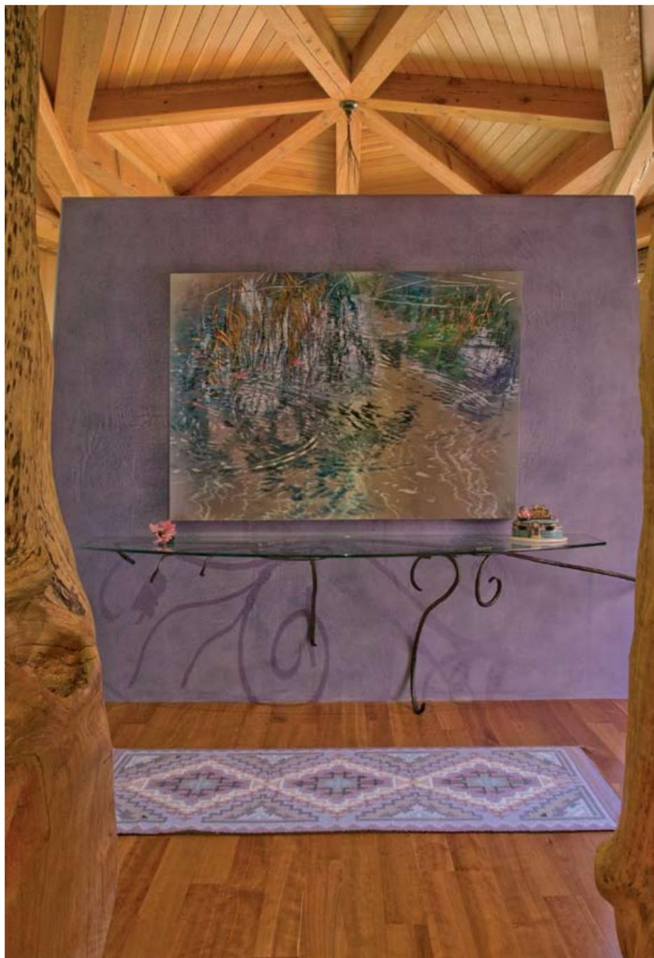
Downplaying its size, the home has a sense of intimacy enhanced by organizing the main living spaces into five "pavilions," each with its own raised ceiling/roof structure. Posts, individually selected then crafted from hand-sanded juniper tree trunks, support sinuous curving wood beams of resawn douglas fir. The perimeter beam detailing is reminiscent of the beams used to construct the roofs of Navajo hogans — with beautiful structural patterns originally inspired by how the Anasazi
