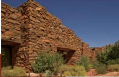
The architects chose local, surface-weathered sandstone to construct the perimeter walls. This stone is laid in a horizontal pattern, echoing the geologic layers and honoring historic cliff dwellings preserved in nearby canyons.
